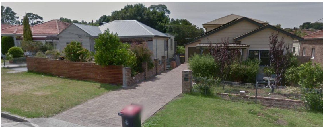
20 and 22 Pheasant Street forming the subject development site
