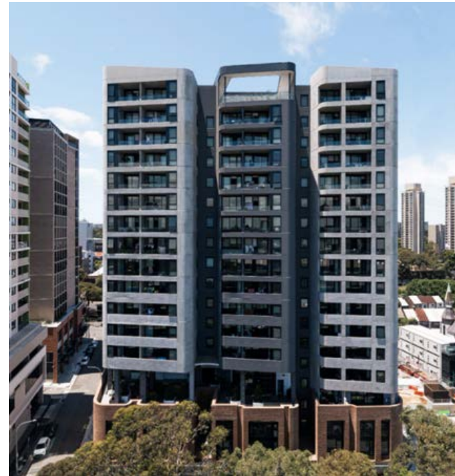
Building mass reduced in scale by creating vertical elements and varying materials and podium and tower levels
