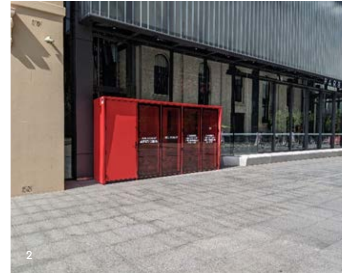
High quality screening used to minimise the visual impact of services on the streetscape and provide an uncluttered and orderly appearance to buildings
